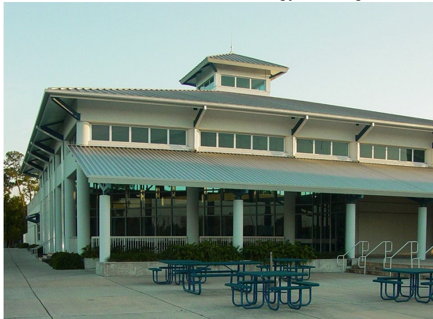
Exterior of TLC showing Cupola
