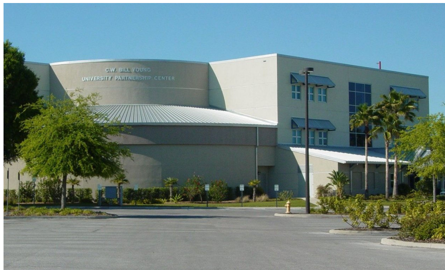
South Entrance to UP from Student Parking Lot
