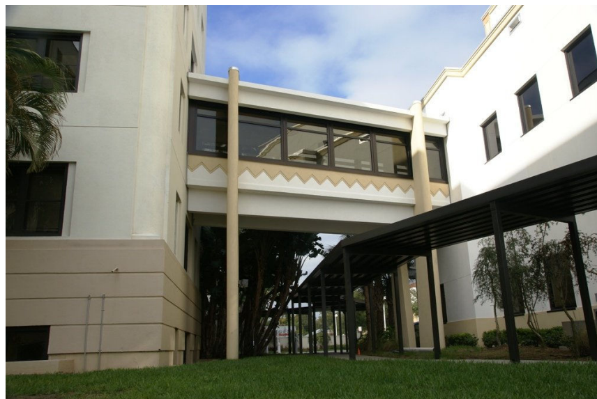
New 2nd Floor Walkway Between Two Buildings
