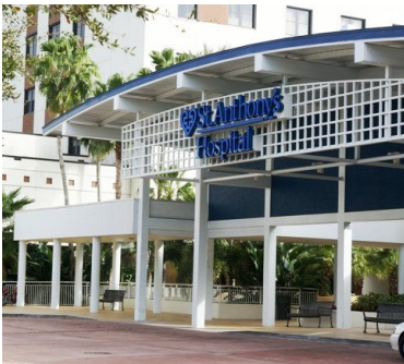
New Entrance Canopy
