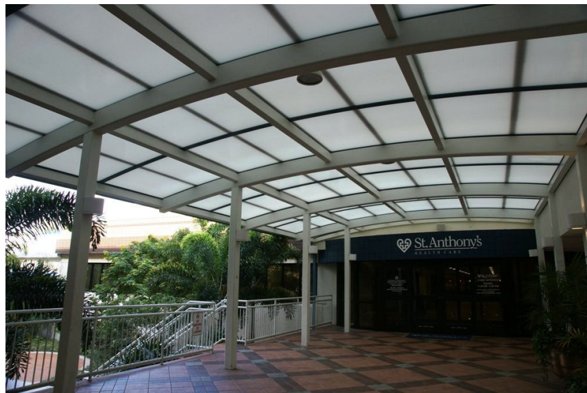
New Covered Terrace Walkway
