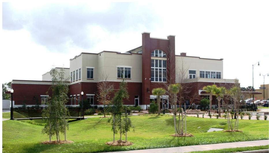
Rear of Leesburg Library
