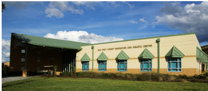
Designed using reinforced masonry supporting Precast concrete roof slabs and long span steel trusses at the Gymnasium. Designed as an Enhanced Hurricane Shelter.
